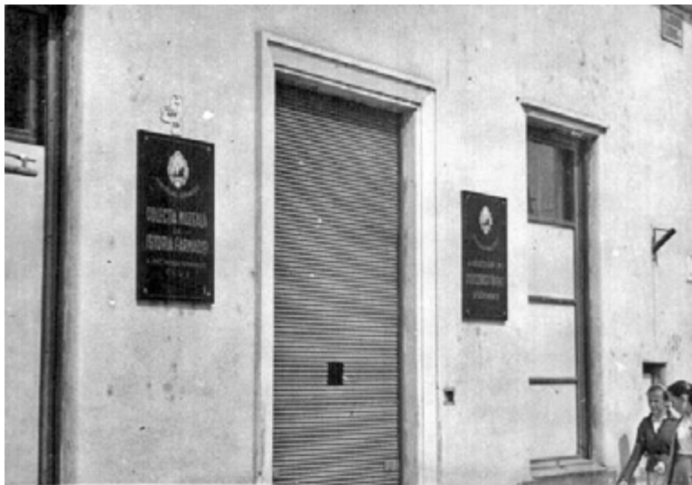
Fig. 5. The entrance to the pharmacy museum (sometime between 1954 and 1959).
