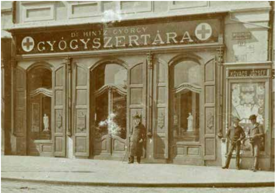
Fig. 8. The entrance to the Hintz House in 1905, detail of a photograph by Ella Hintz.
